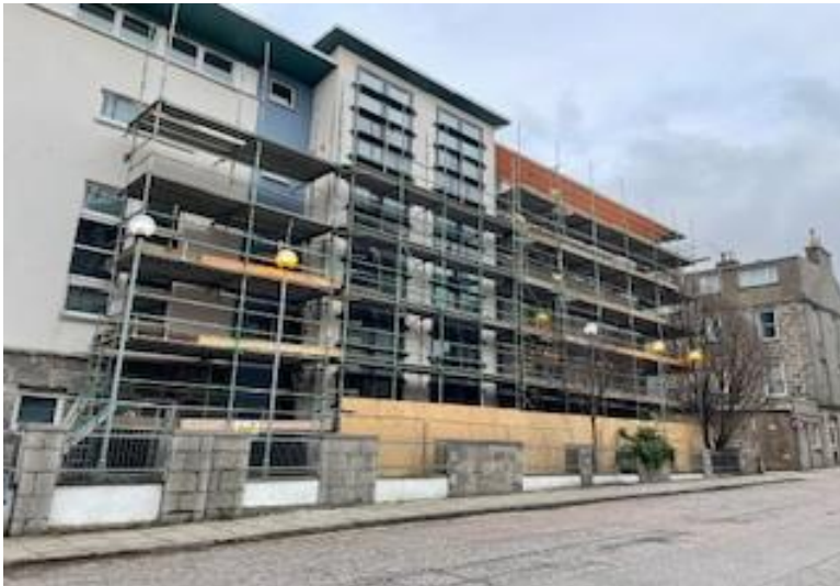
Phase 3 Scaffolding ongoing
