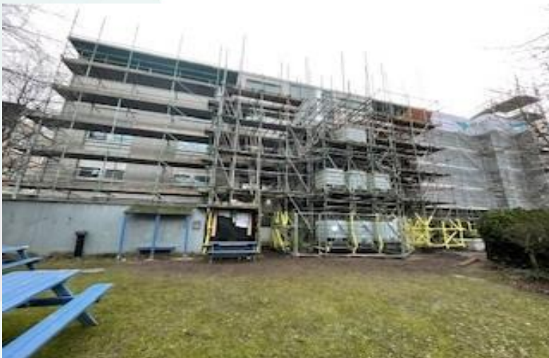
Phase 2 scaffolding ongoing
